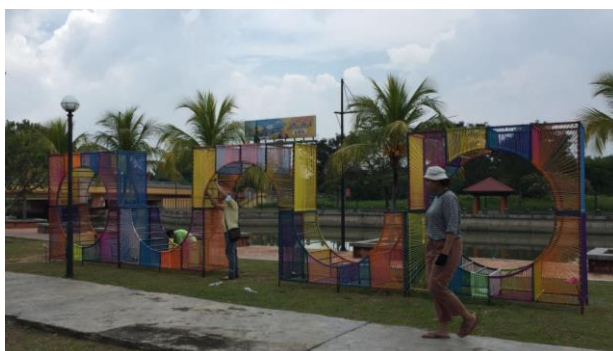
Figure 5 Careful Wiring Begins after Artwork Assembly (Photo Credit: Suzy Sulaiman)
